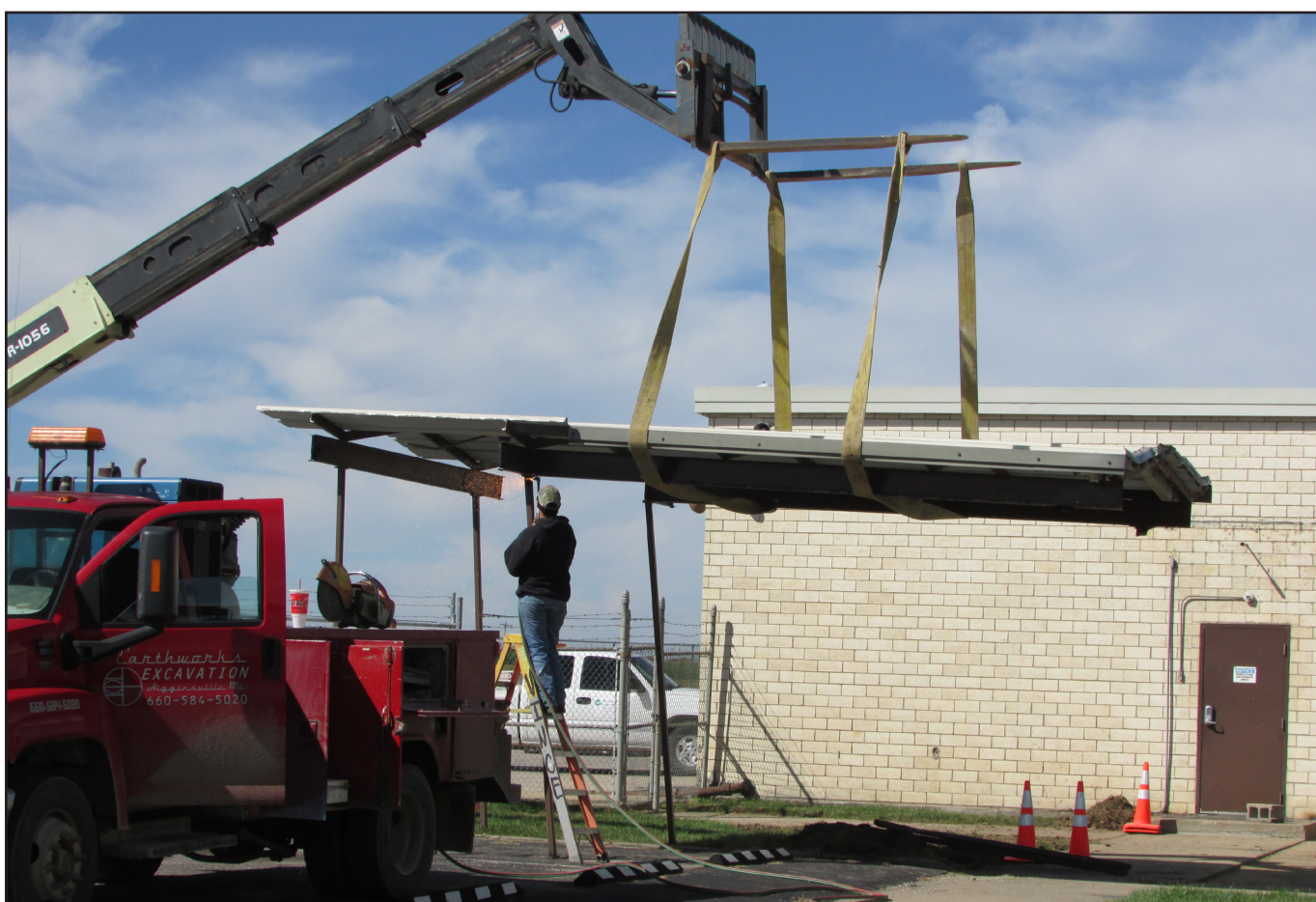
Contractors remove a portion of the old awnings covering the sidewalks of the employee entrances to WCE's headquarters building.
